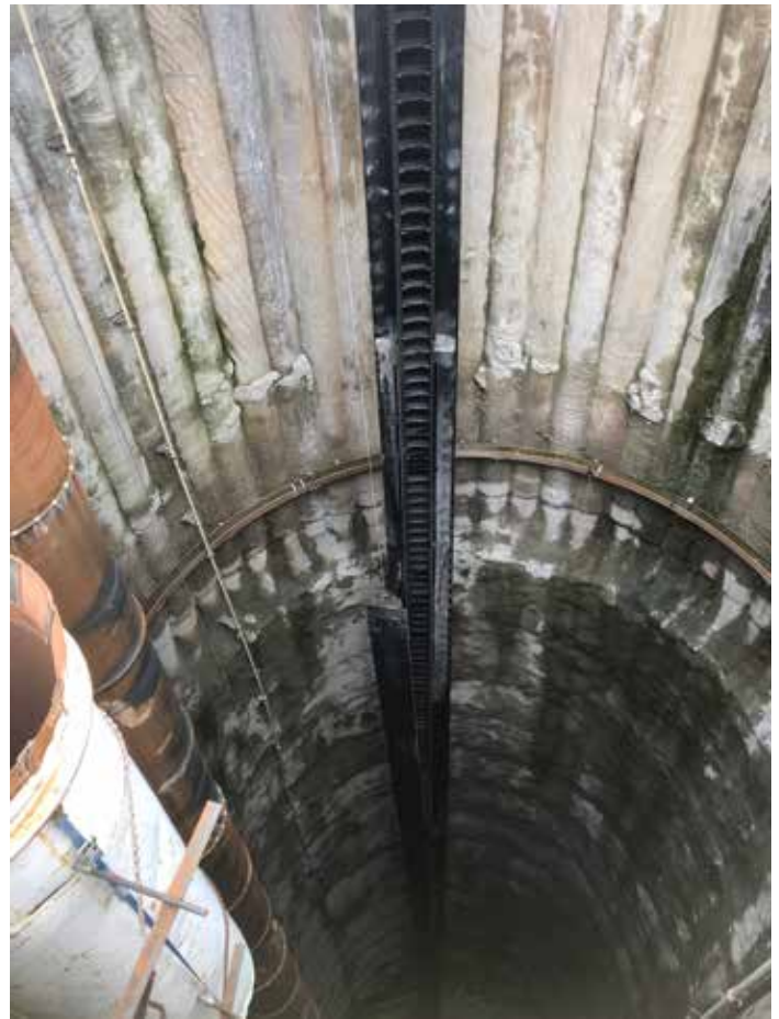
The tunnel's working shaft allows access and ventilation for workers 18 stories underground.
