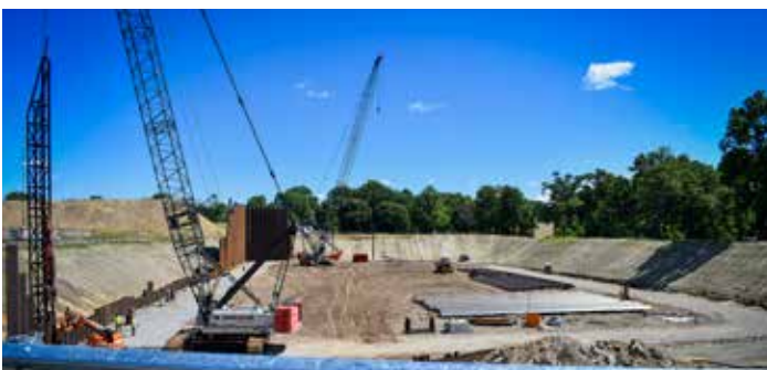
In June 2017, excavation of the basin was underway.
