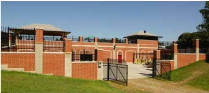
The control building for the Shawnee Park CSO Basin is built into the hillside. There is a new pavilion and restrooms built on top.
