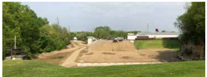
April 2019, Clifton Heights Basin construction is complete and the basin is covered with 12 feet of dirt.
