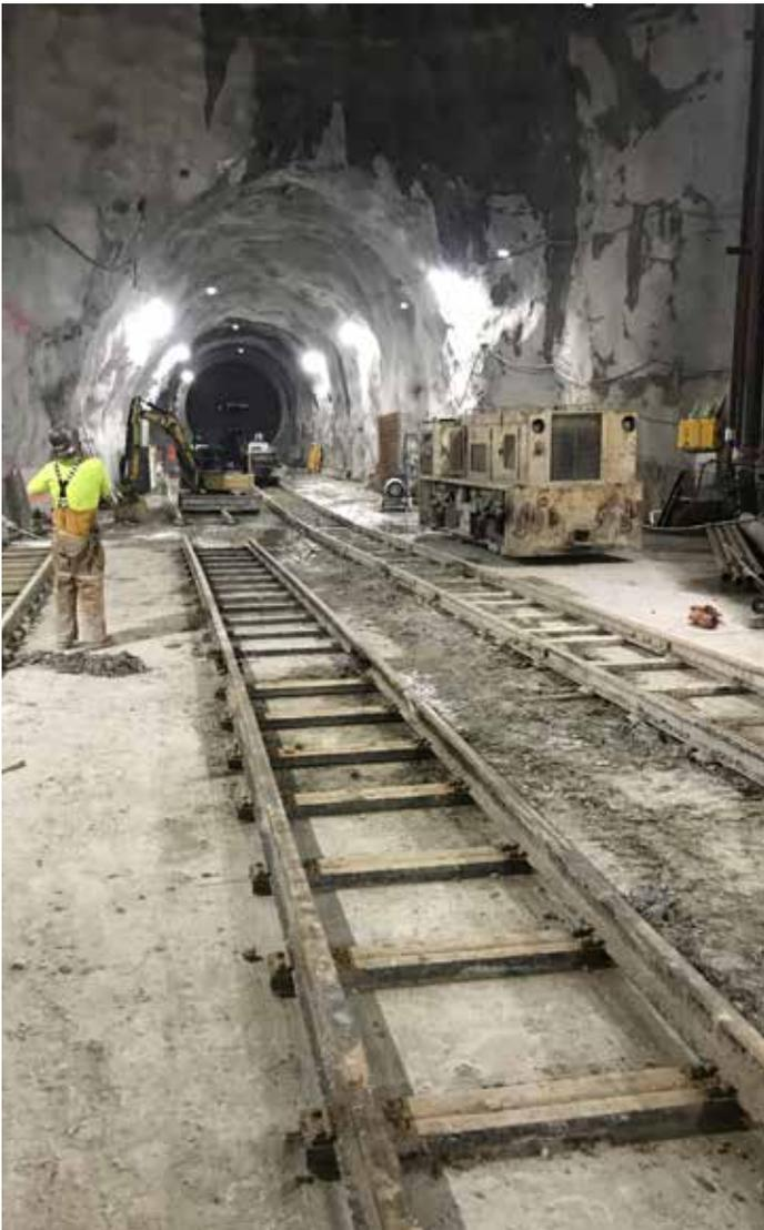
Crews work to install a rail line to transport both workers and rock through the tunnel.
