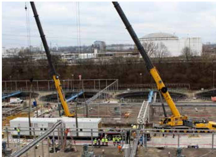
Cranes place a new oxygen generation component in place.
