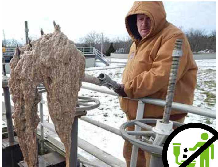
A large wiper clog is dislodged at our Hite Creek Water Quality Treatment Center
