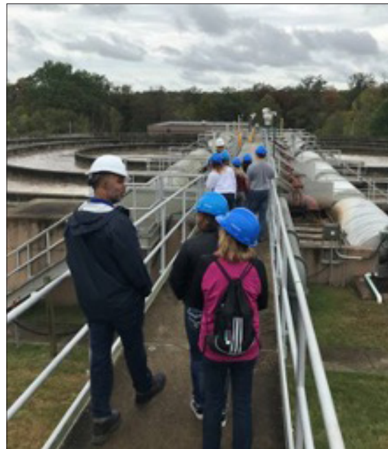
MSD’s Floyds Fork Water Quality Treatment Center
