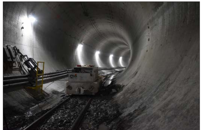
Waterway Protection Tunnel
