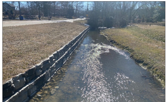
Mount Holly bank stabilization
