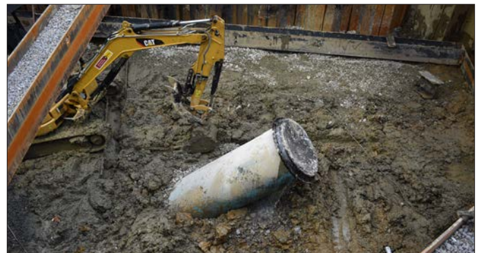
Harrods Creek sewer repairs
