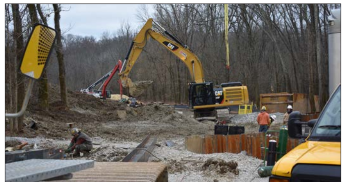
Shaft to access break along Harrods Creek
