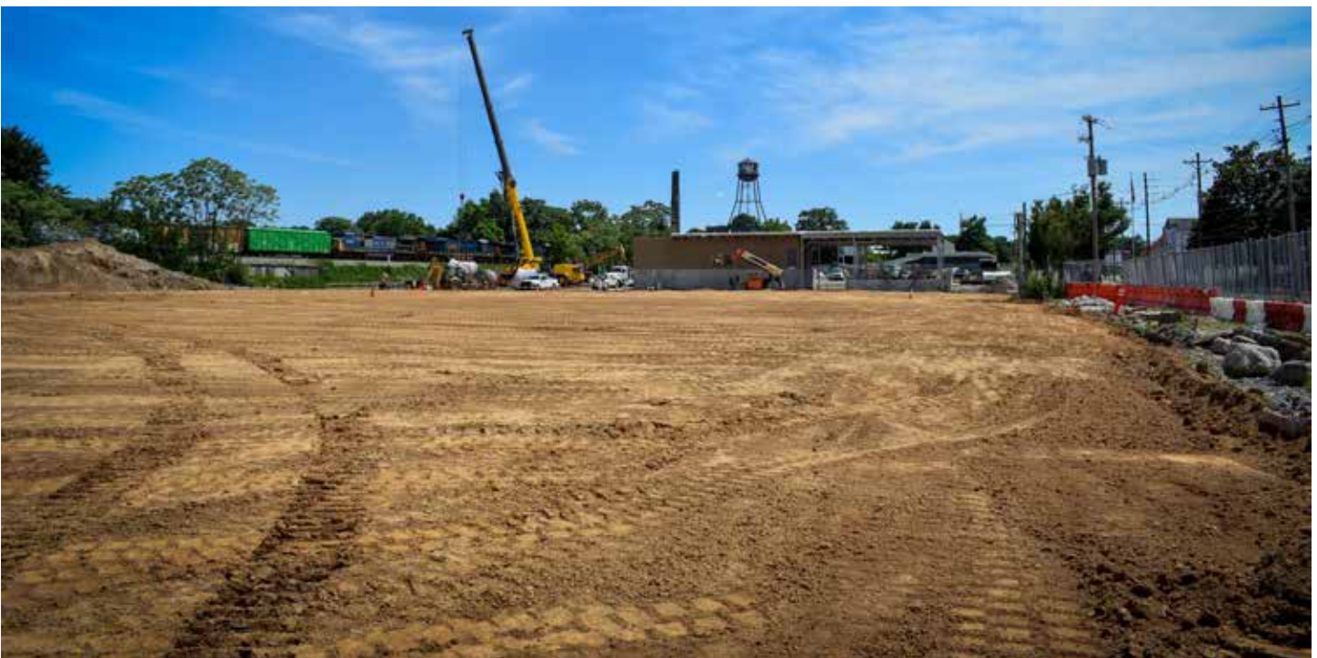
Below: Soil is leveled on the roof of the Logan CSO Basin.
