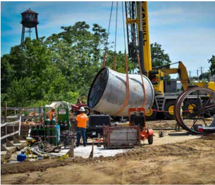
Above: A crane lifts a piece of the Logan CSO Basin interceptor pipe.
