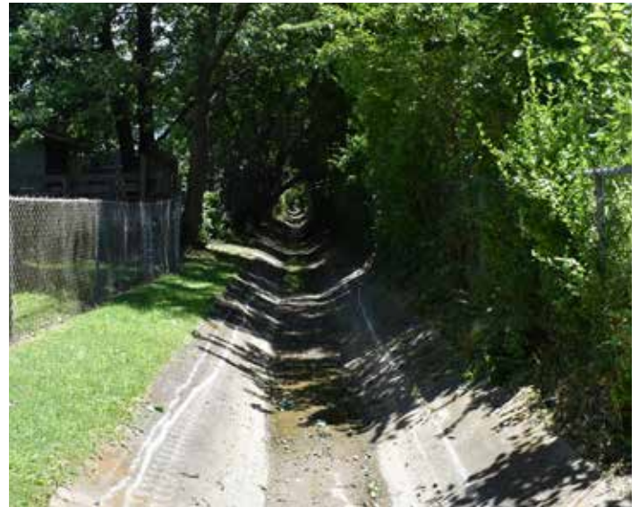
Left, an MSD crew member works to clear plant growth that has obstructed the flow of stormwater. Above, is the newly cleared channel.
