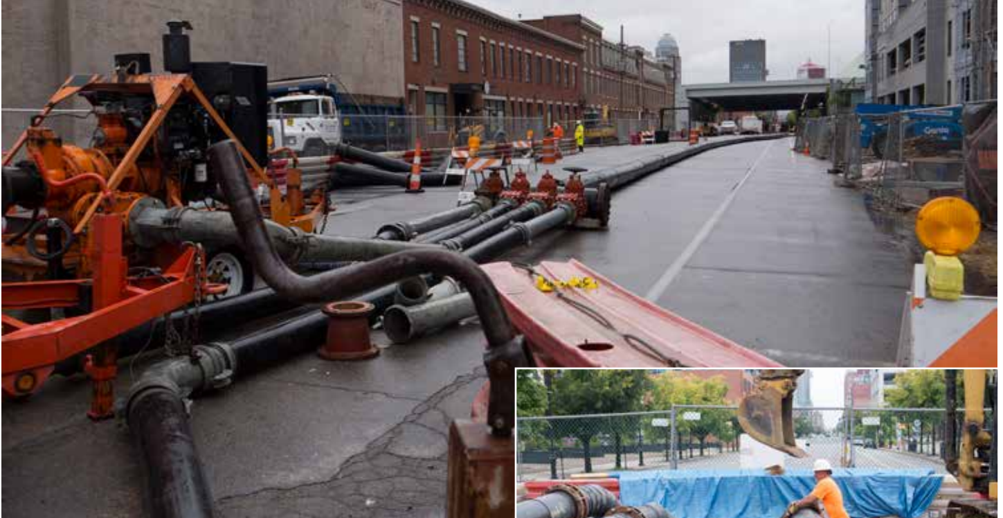
Above: One of the three 18-inch temporary sewerlines is in place.
