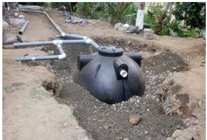
Above, left to right: David Glenn, Trish Capito and Steve Blanford pose with the septic tank prior to installation in Orosi Valley, Costa Rica. Below: Installation of the septic tank and receiving lines are underway.
