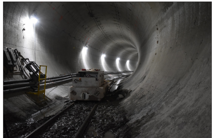
Waterway Protection Tunnel
