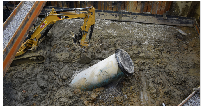
Harrods Creek sewer repairs
