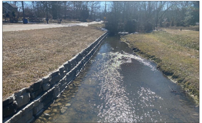
Mount Holly bank stabilization
