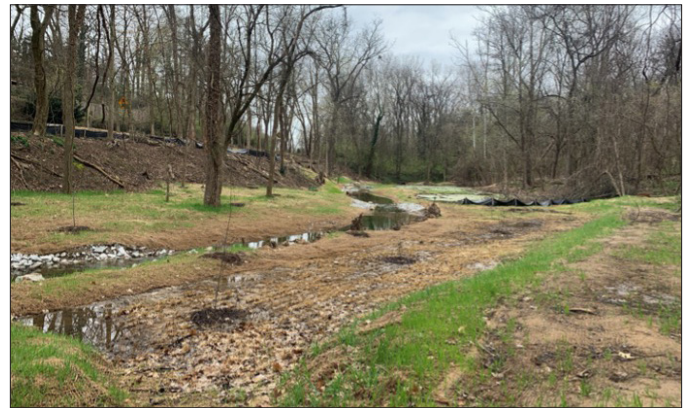
South Peterson environmental restoration project
