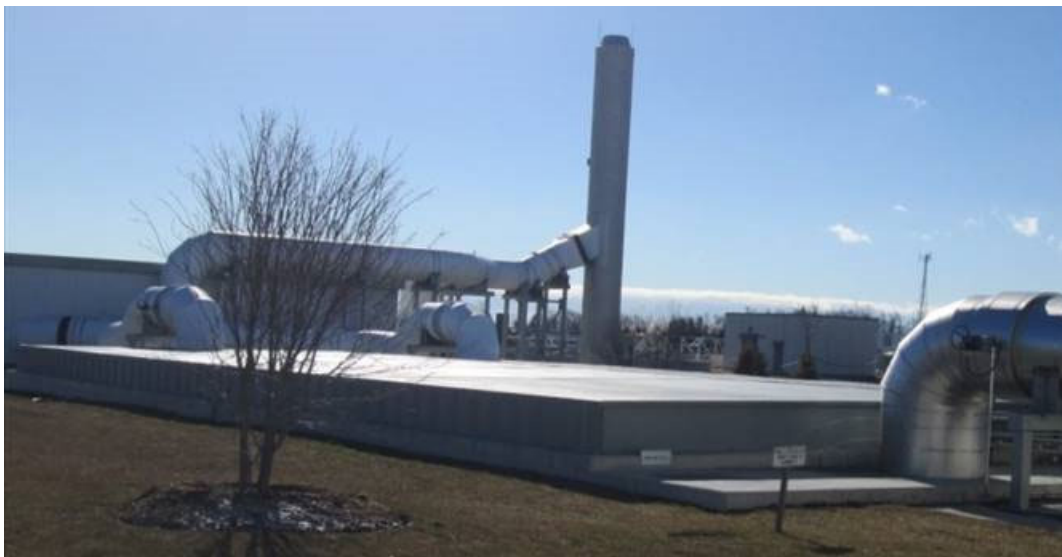
Figure 2 – Example Biofilter Configuration
