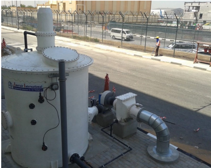
Figure 1 – Example Carbon Adsorption System (Amer Air Intl)
