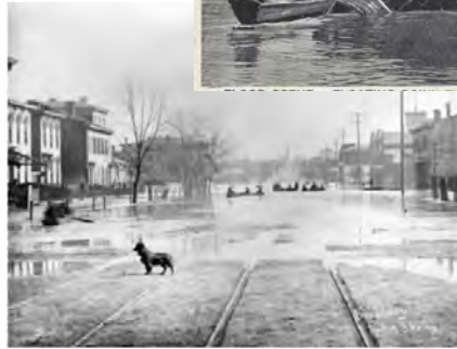
1884 Flood along Broadway east of Shelby Street
