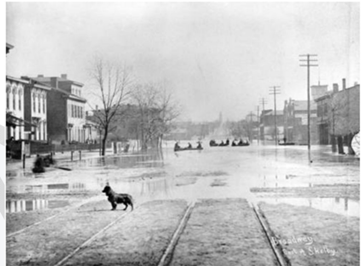
1884 Flood along Broadway east of Shelby Street
