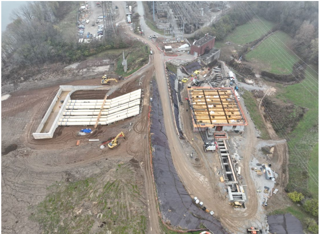
Construction underway at Paddy's Run Flood Pump Station. The original pump station was placed into service in 1953. It provides critical flood protection in addition to serving as an essential wastewater infrastructure for combined sewer overflow control.
