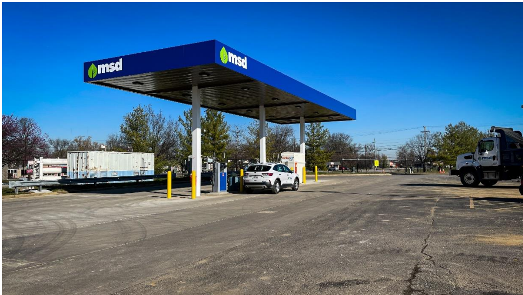
MSD's Central Maintenance Facility
