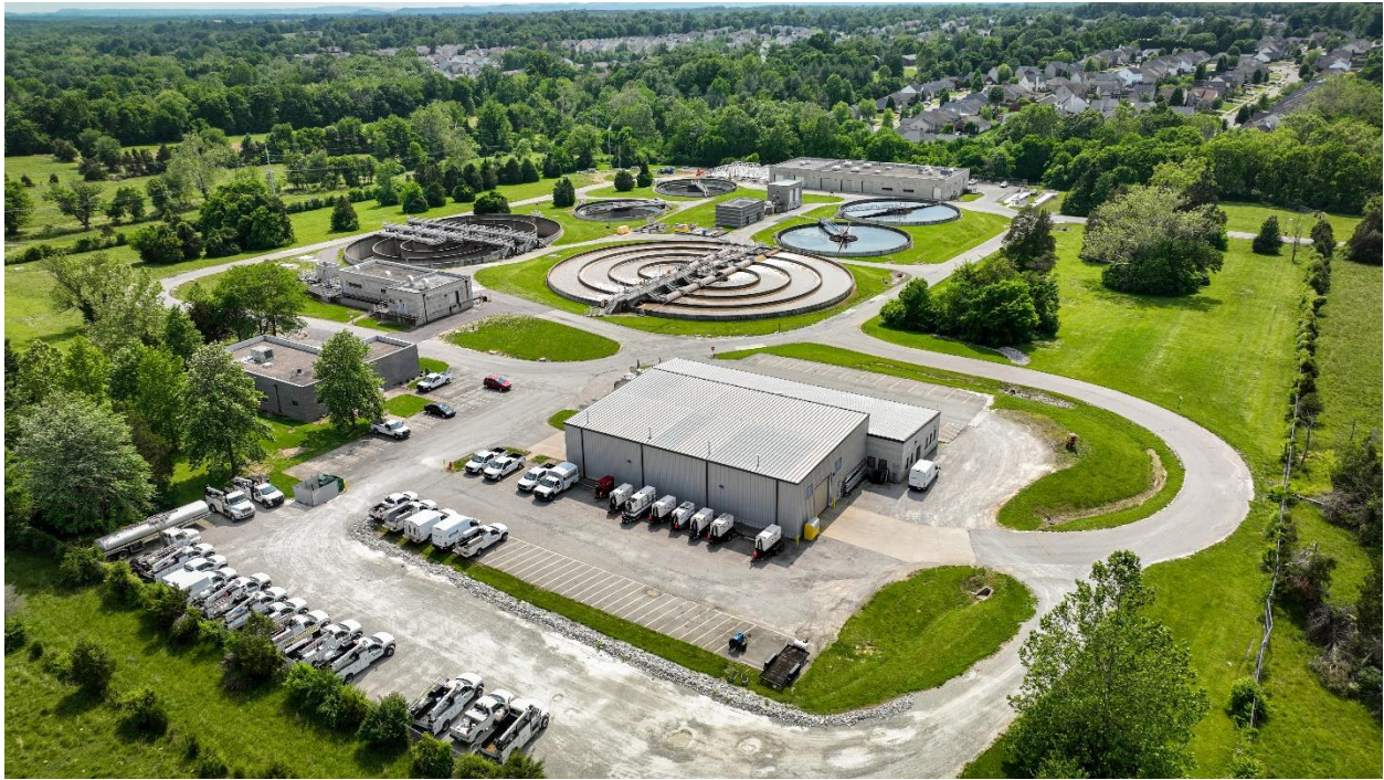
MSD's Cedar Creek Water Quality Treatment Center
