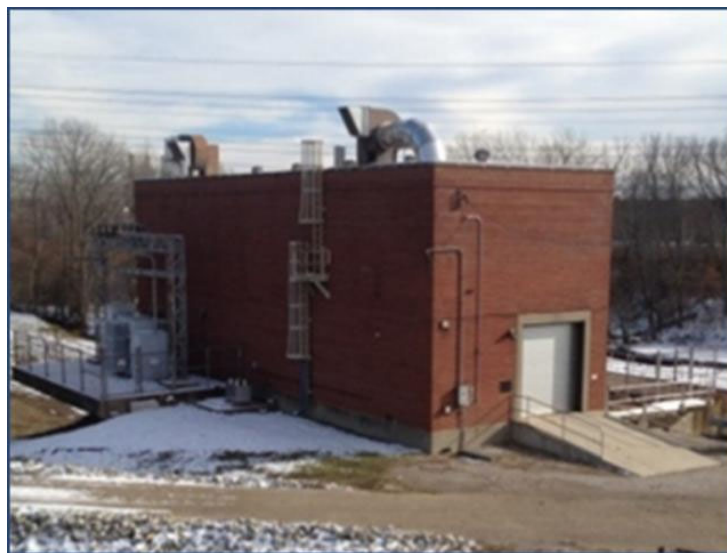
MSD's Paddy's Run Flood Pump Station, constructed 1953.
