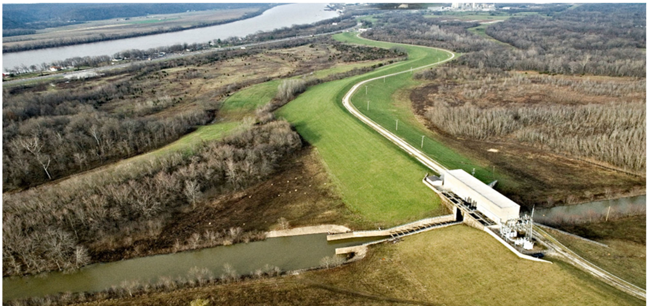
MSD's Pond Creek Flood Pump Station
