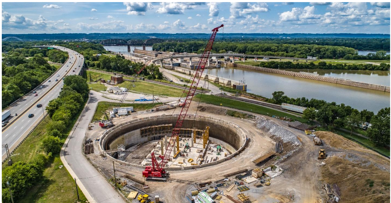
MSD's Portland Combined Sewer Overflow Basin
