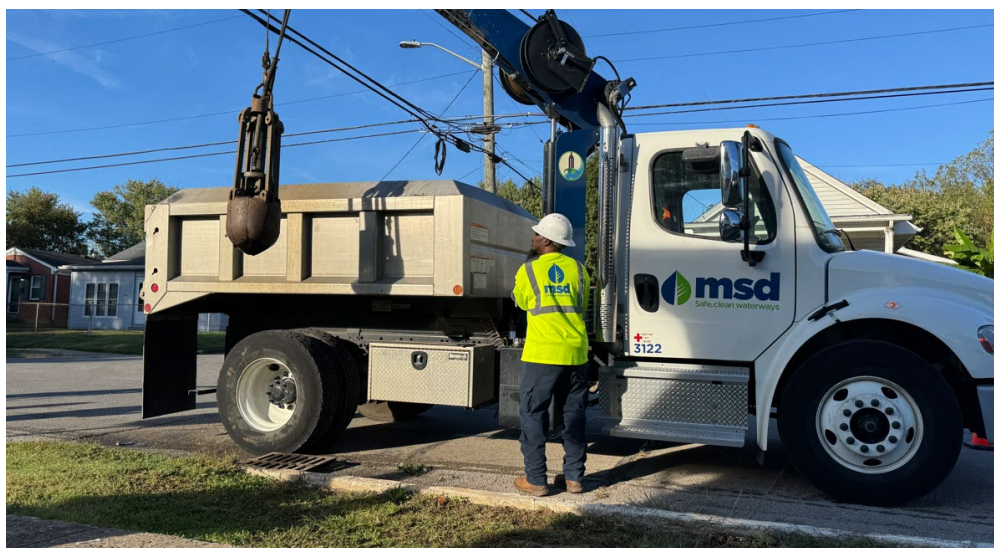
Utility Worker cleaning a catch basin as part of odor control work.
