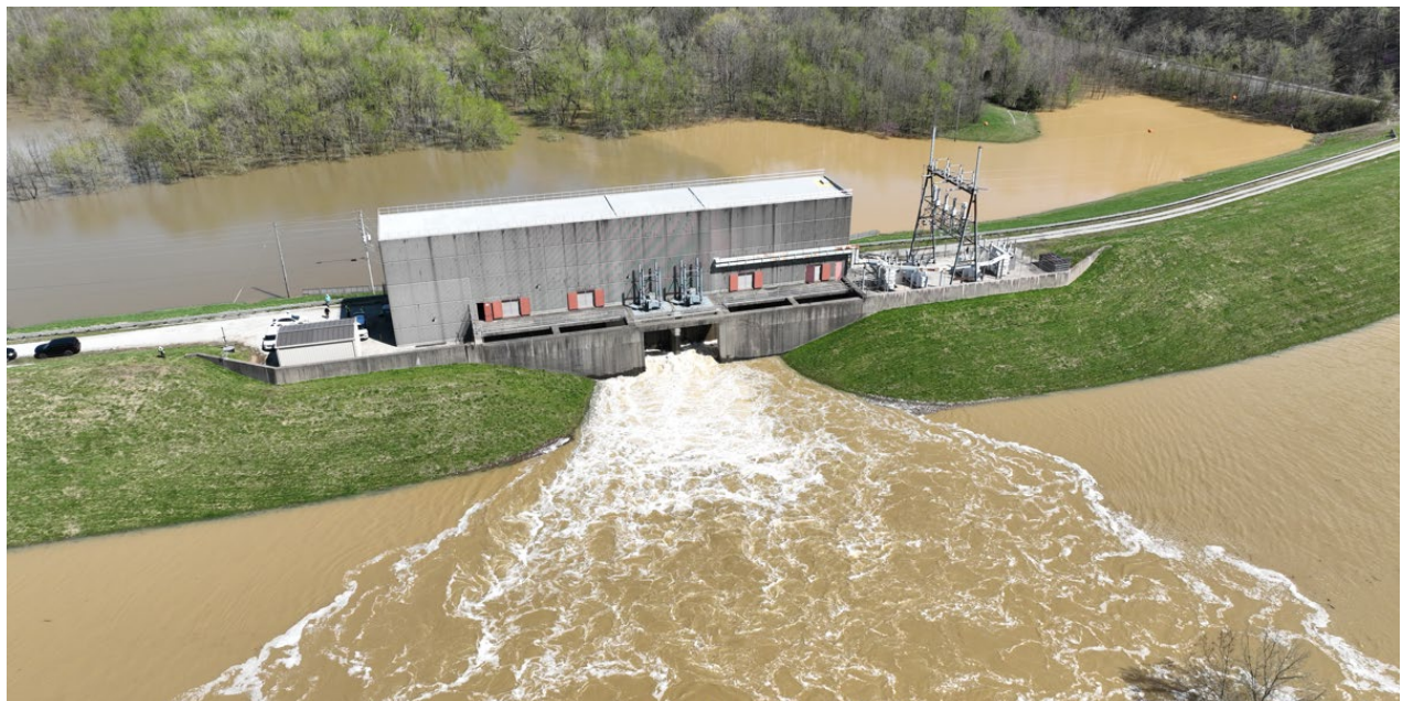
Pond Creek Flood Pump Station in operation during a flooding event.
