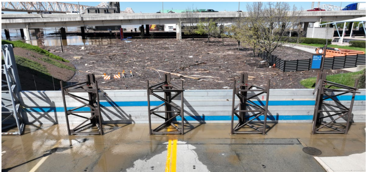
A portion of the floodwall that MSD crews erect to protect downtown Louisville from a rising Ohio River.
