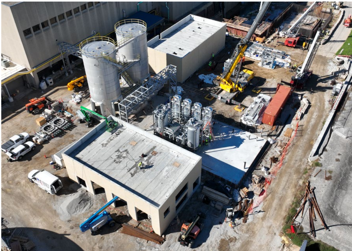
Construction at the Morris Forman WQTC biosolids facility.
