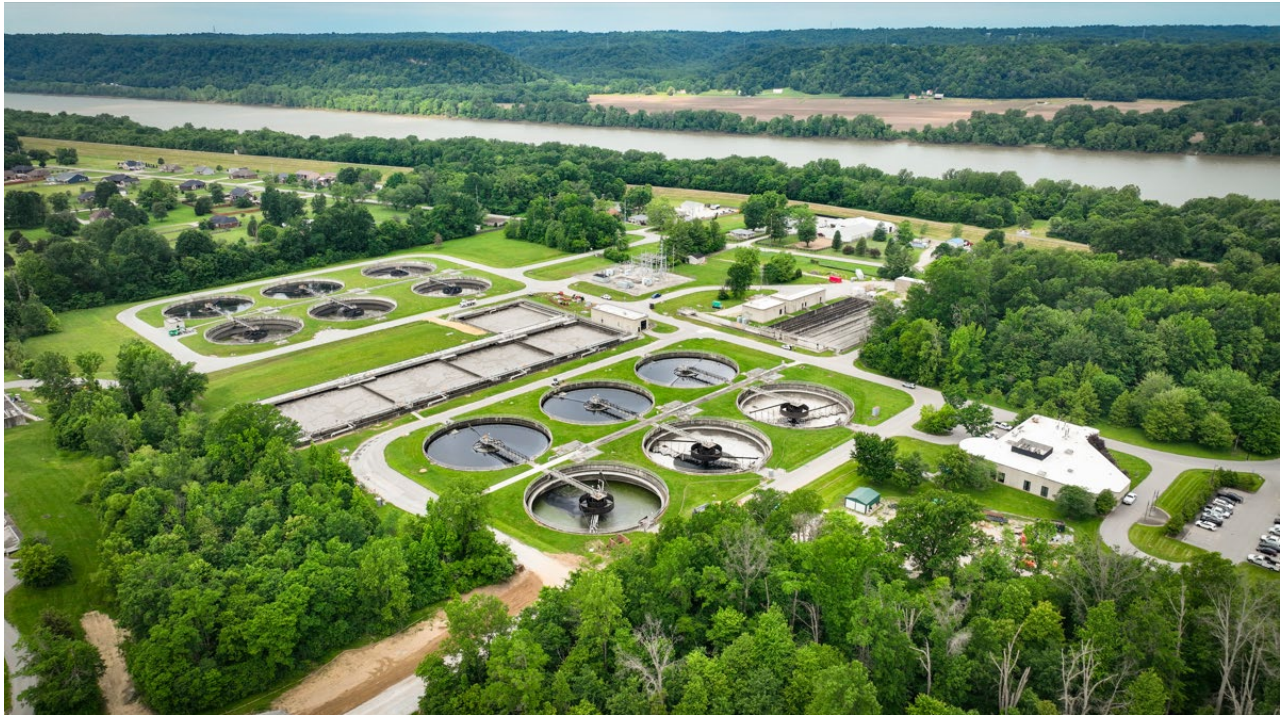
Derek R. Guthrie WQTC located in southwestern Jefferson County.
