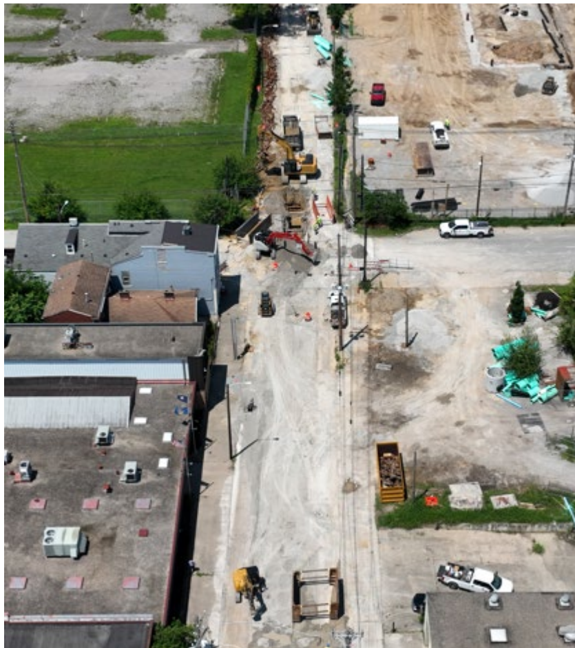
Emergency sewer line replacement on East Liberty Street of a brick sewer dating back to 1872
