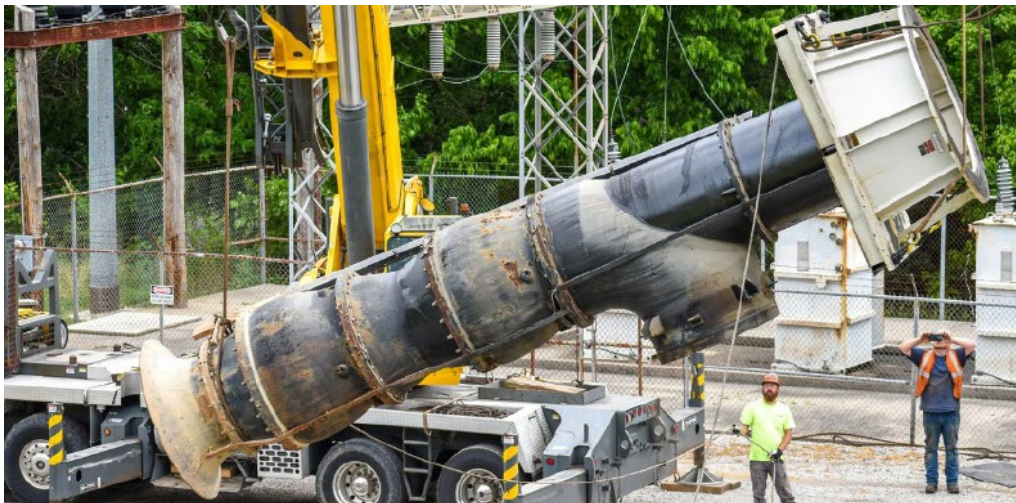
A 1,120-horsepower pump and motor from Lower Mill Creek Flood Pumping Station was shipped to Kansas City to be rebuilt after damage sustained during the April Flood in Louisville
