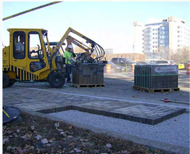
Mechanical installation of permeable interlocking concrete pavers
