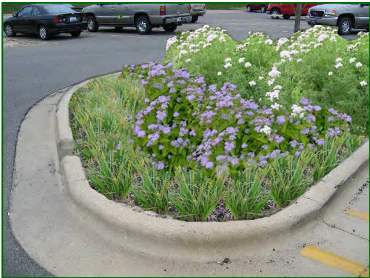
Typical parking lot bioretention cell shown during mid-summer blooming season (Concept Rendering: Margaret Shea & Shea Powell, Dropseed Nursery)
