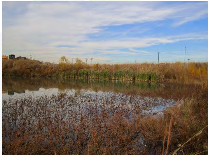
Constructed wetland cell in Buechel
