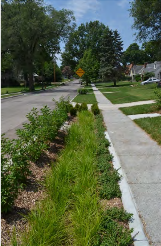
Native and Cultivar plants used in a residential rain garden. (Photo: David Dods, URS)
