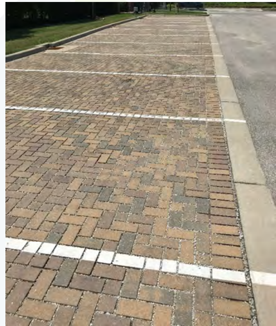
Permeable Pavers at Brown Foreman
