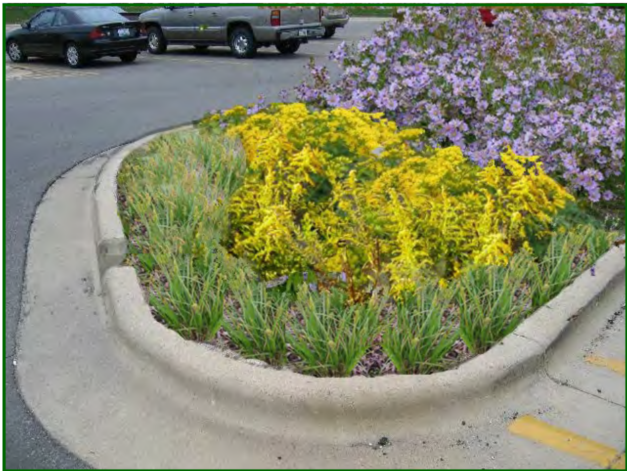
Typical parking lot bioretention cell shown during fall blooming season (Concept Rendering: Margaret Shea & Shea Powell, Dropseed Nursery)
