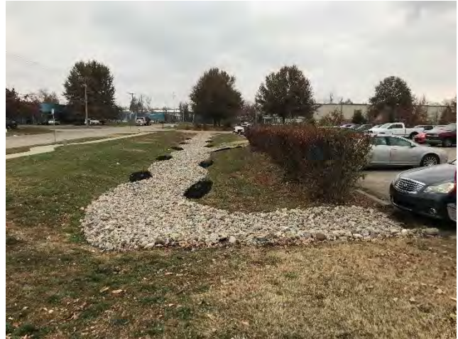
Open Infiltration Trench at Misa Metal Fabricating, Inc.
