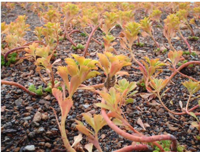
Sedum being used in a green roof application (Photo: Courtesy of The Green Building)
