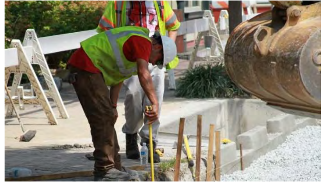
Construction of permeable paver parking lane and tree boxes
