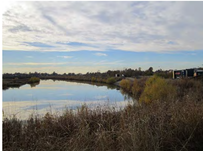
Green Wet Basin in Buechel has a naturalized buffer
