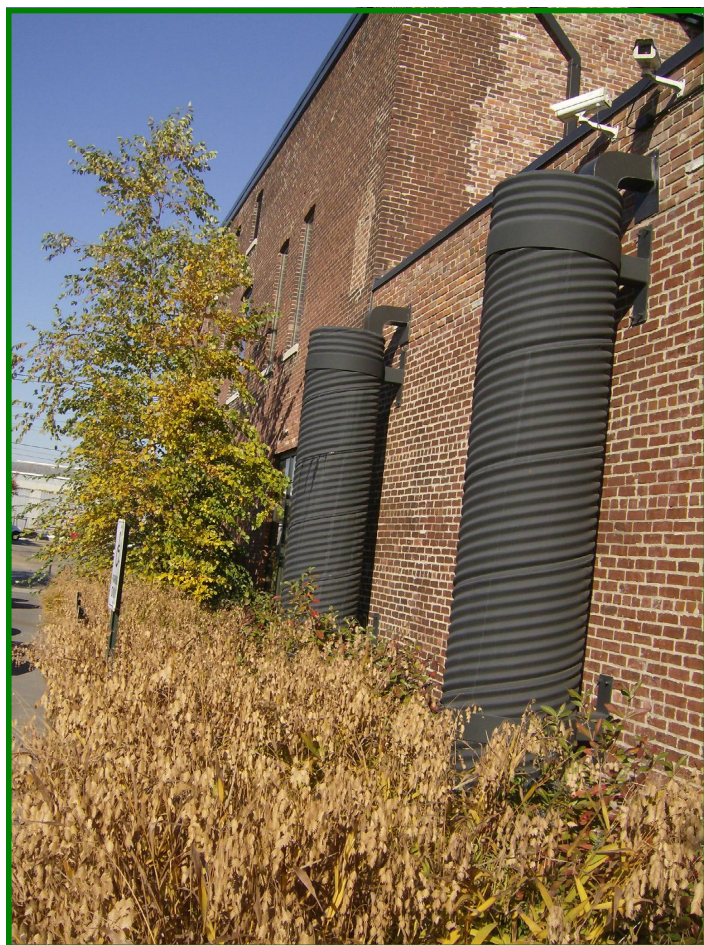
Cisterns harvest rainwater and water the rain gardens below at the Green Building
