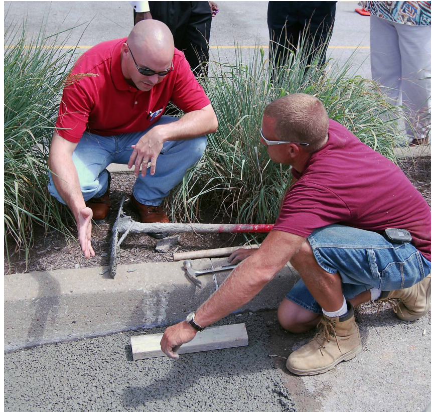
Installation of Pervious Concrete
