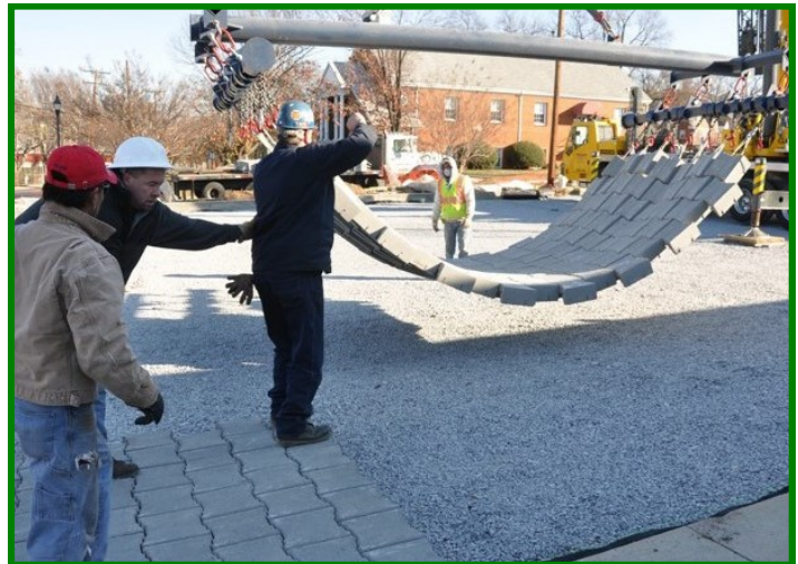
Installation of permeable articulated concrete block mats
