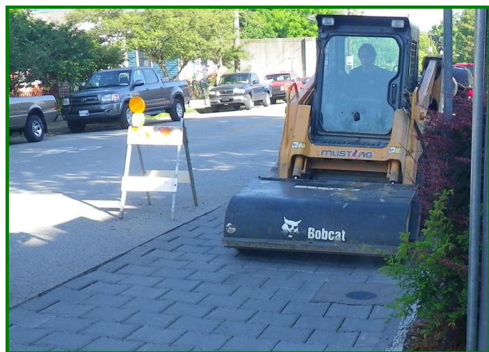
Cleaning of permeable pavers
