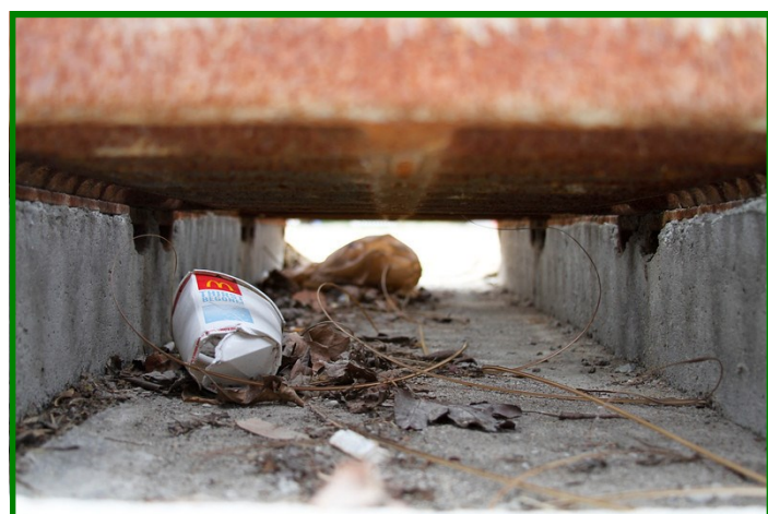
Infiltration Trenches should be cleaned and kept free of dirt, trash, and debris
