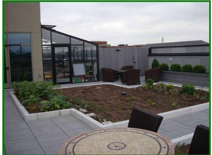
Roof garden patio includes a green house and extensive green roof planted with vegetables and herbs
