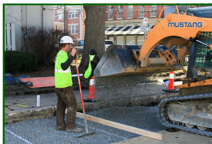
A contractor applies aggregate for placement of permeable pavers
