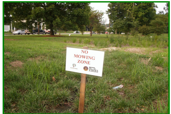
“No Mow” maintenance signs installed at a rain garden in a Louisville Metro Park
