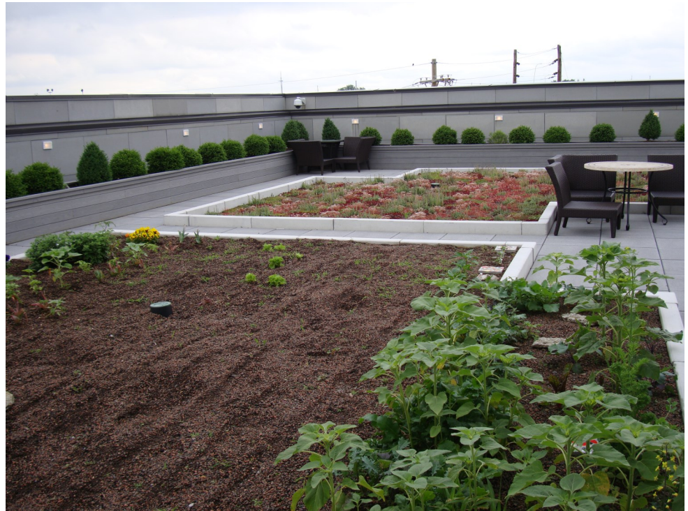
Extensive green roof planted with vegetables (foreground) and sedum (background)
