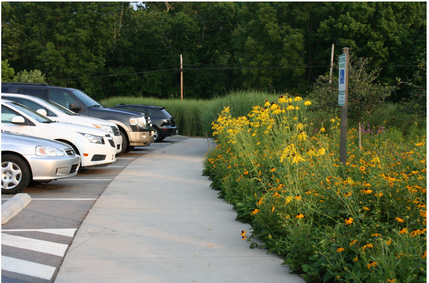
Parking lot runoff drains to a vegetated buffer at the Parklands of Floyds Fork
