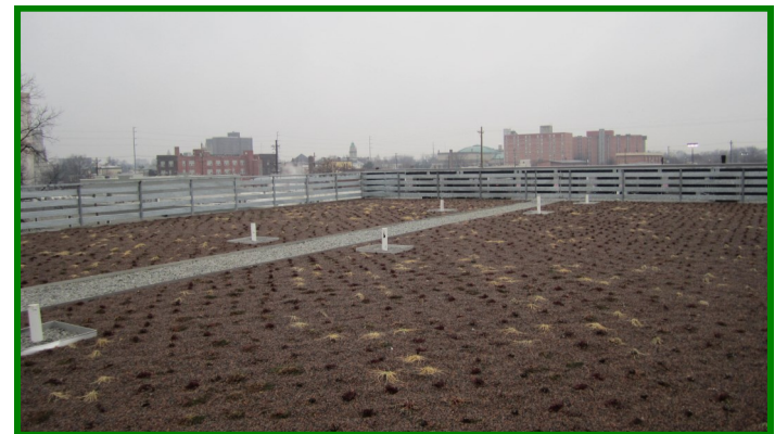
Extensive green roof with non-vegetated access path and buffers around vents
