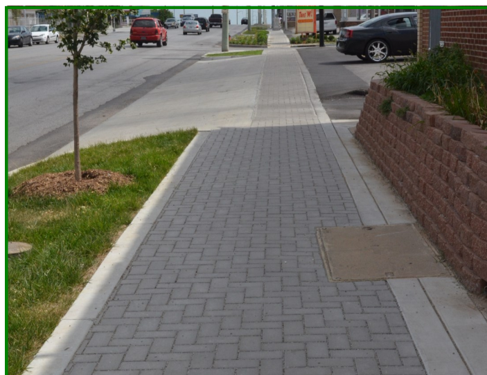
Permeable pavers should be kept free of dirt and debris
