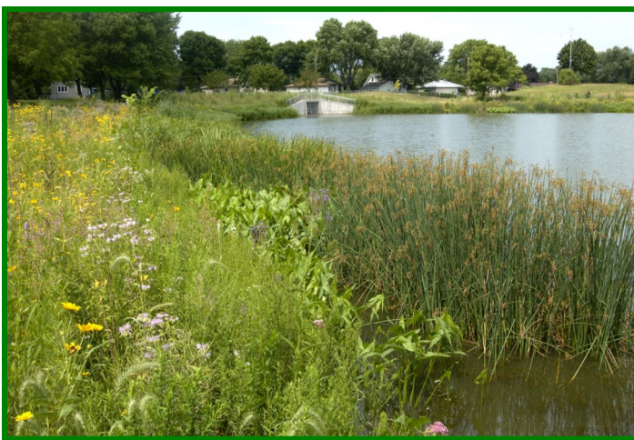
Wet basin with native vegetation along the perimeter. Trash and debris should be removed from practice
