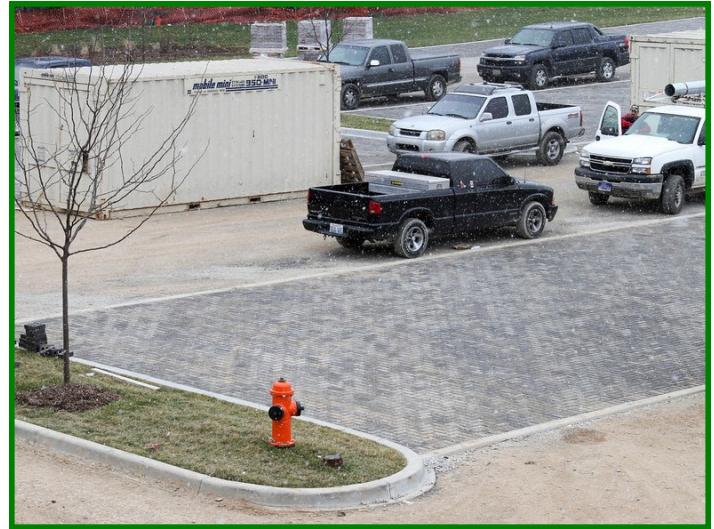
Construction of a green parking lot
