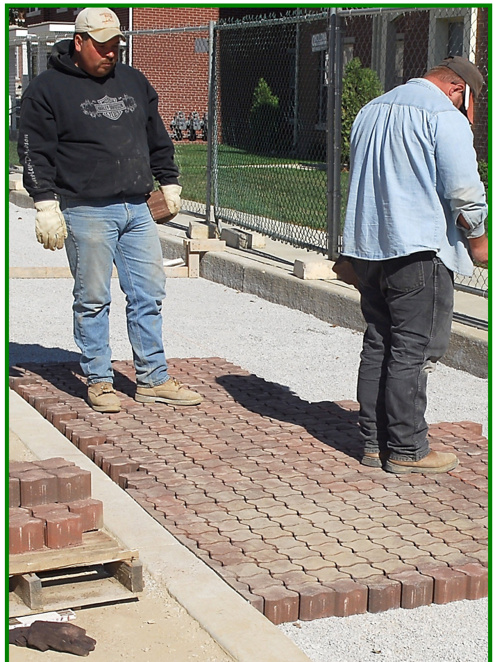
Installation of permeable interlocking concrete pavers
