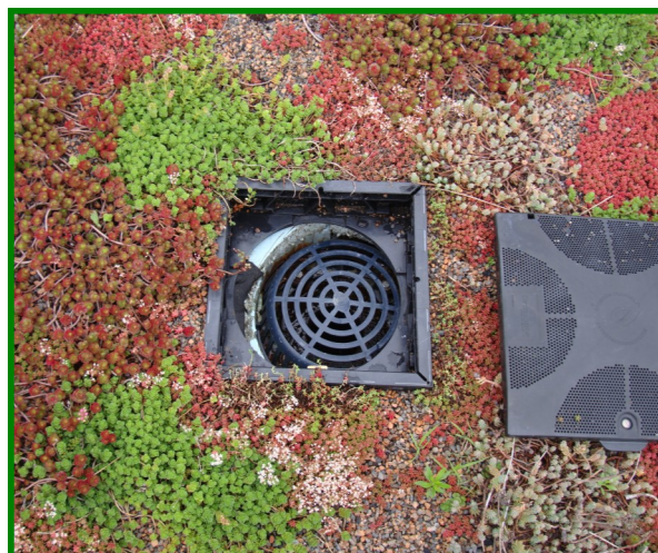
Established sedum plants on extensive green roof
