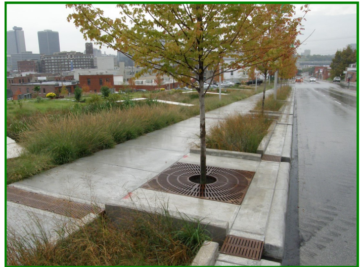
Series of tree and planter boxes accept stormwater runoff from a roadway
