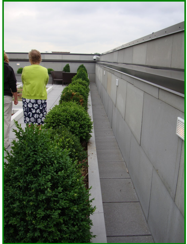
Intensive green roof beds, planted with evergreen shrubs
