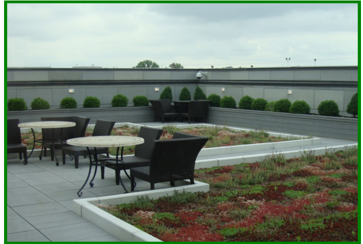
Extensive green roof beds (foreground) are paired with intensive green roof beds (background), planted with evergreen shrubs
