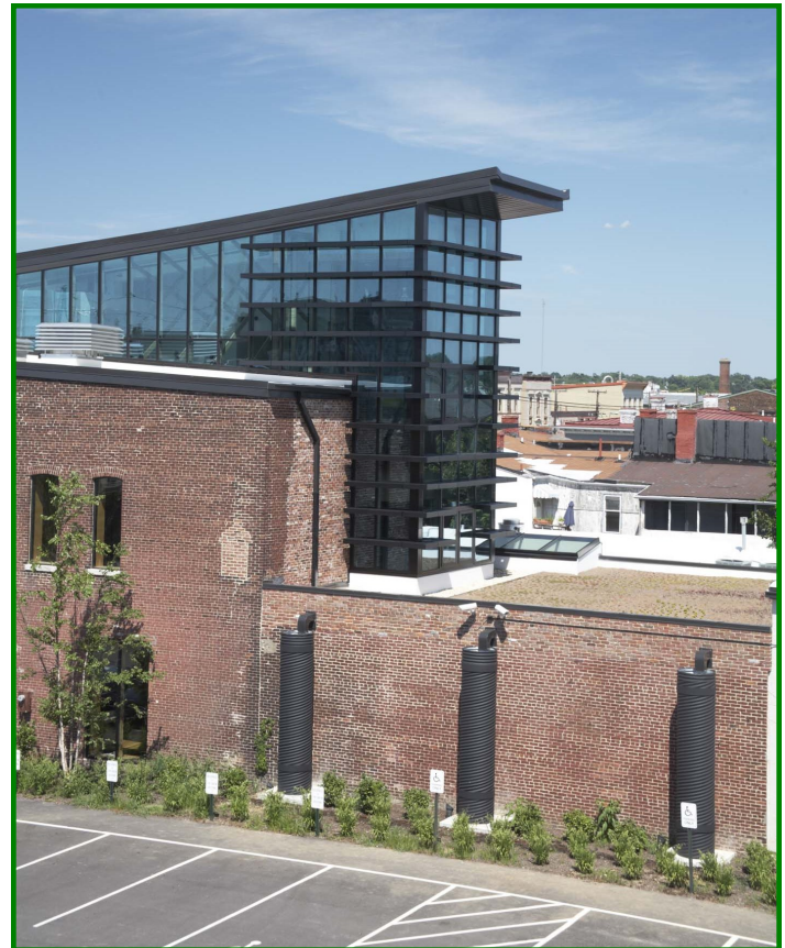
Three cisterns capture and store excess runoff from rooftop surfaces at the Green Building and are drained between rain events to water the bioswale and rain garden.
