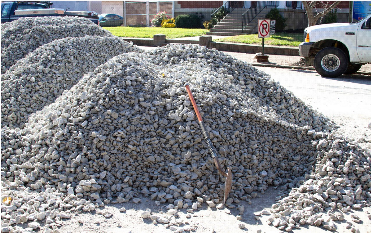
Stone used as a base layer for Green Infrastructure
