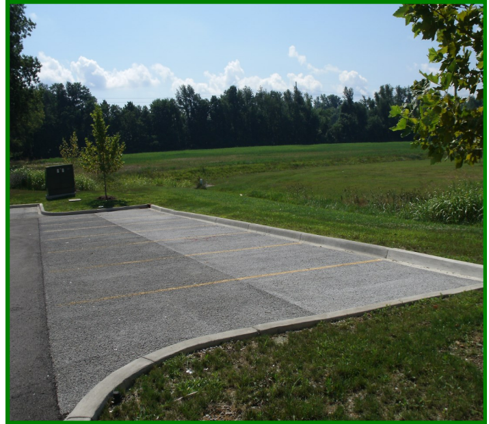
Pervious Concrete Parking Spaces
