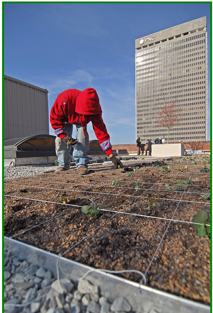
Installation of plants on an extensive green roof
