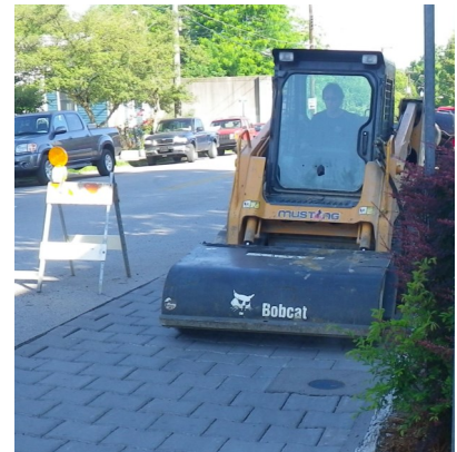
Clockwise from top left: number 8 Stone into permeable pavers, cutting back old growth on native plants, mulching a rain garden, sweeper removes dust and debris from pervious pavers.
