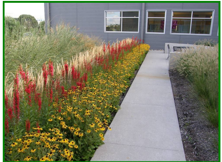
A linear rain garden, or bioswale, conveys stormwater runoff from the building's downspouts
