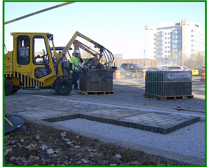
Mechanical installation of permeable interlocking concrete pavers
