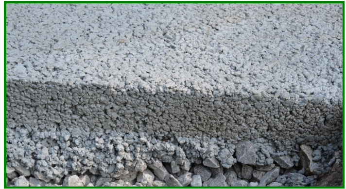
Pervious Pavements should be kept free of dirt and debris to keep the practice draining effectively
