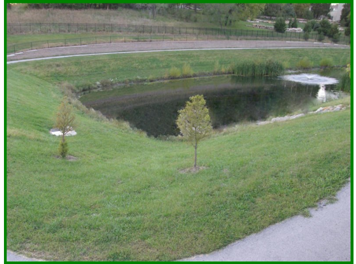
Wet basin with small buffer
