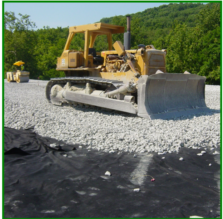
Construction of Porous Asphalt
