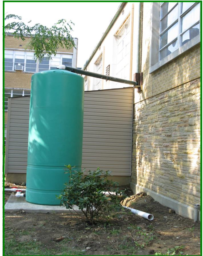
Cistern under construction
