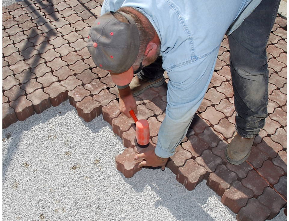
Installation of permeable interlocking concrete pavers
