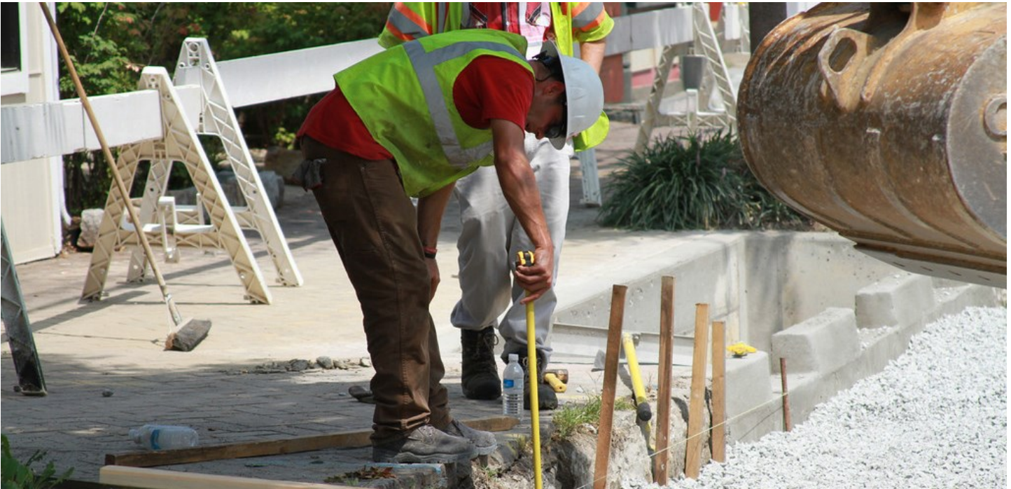
Construction of permeable paver parking lane and tree boxes
