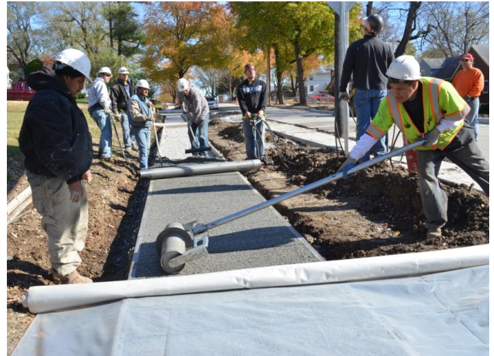
Construction of a pervious concrete sidewalk
