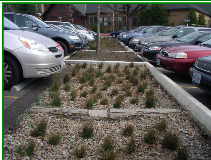
Linear rain garden/bioswale with rustic log check dams
