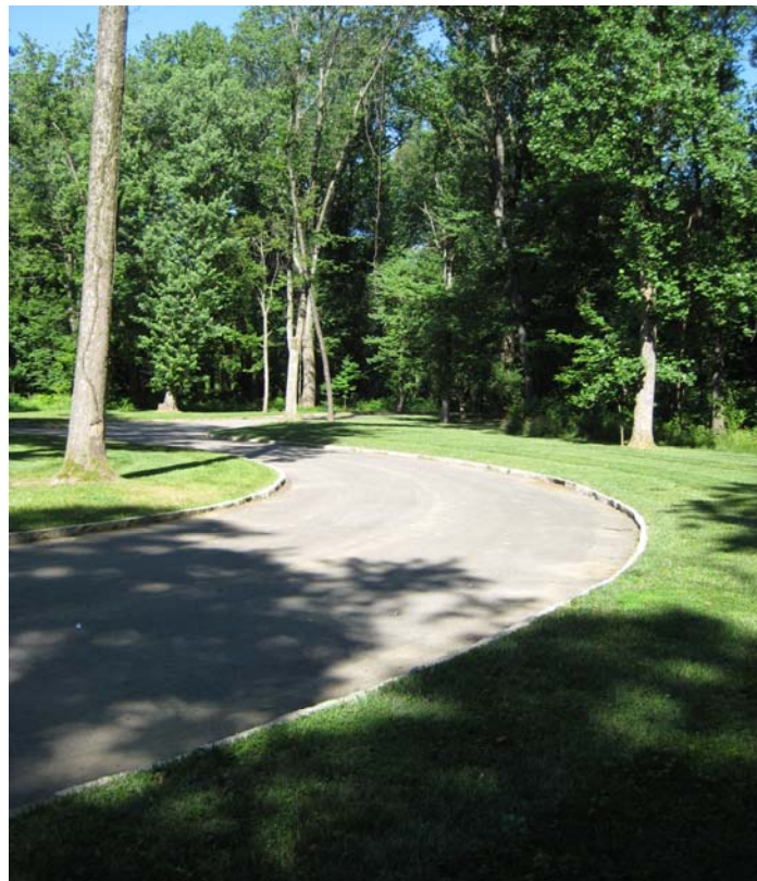
Figure 18.2.4-F. This residential street in a development using conservation and open space design uses narrower streets than traditional practices.
