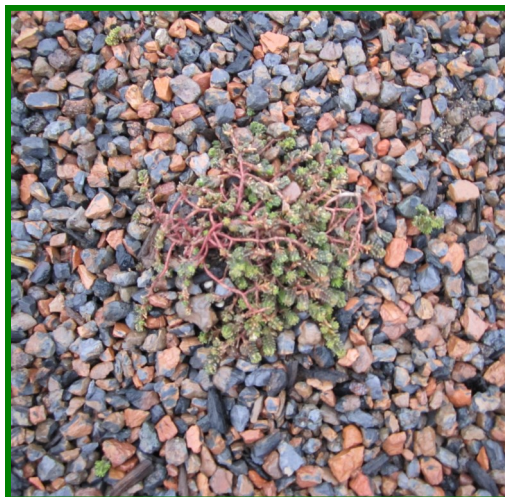
Newly planted sedum on extensive green roof
