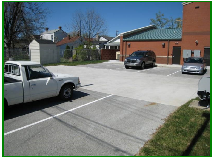
Pervious concrete at Louisville Fire Station
