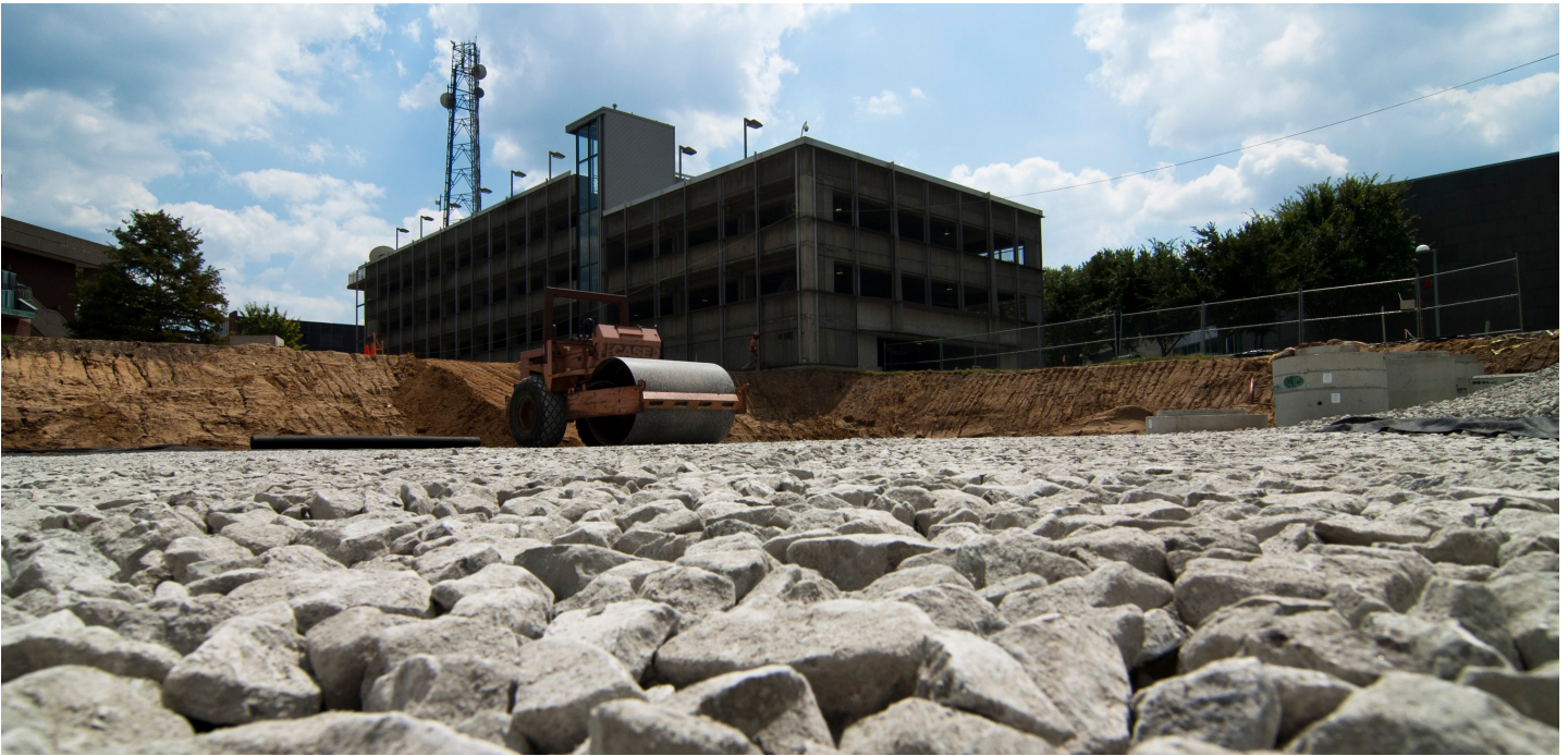
Construction of infiltration basin at the University of Louisville
