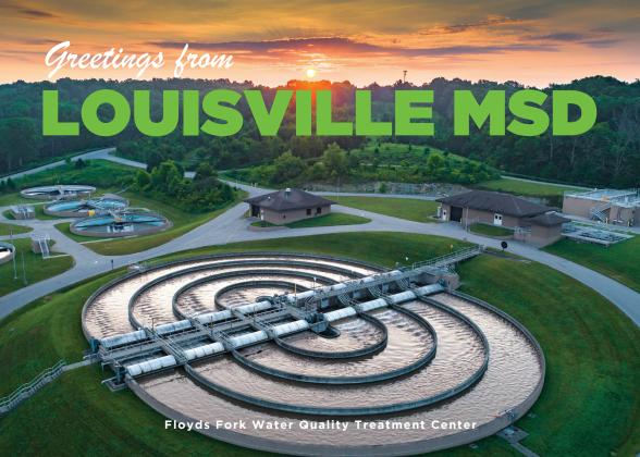
Floyds Fork Water Quality Treatment Center receives an average of 3.5 million gallons of wastewater per day. Here, wastewater goes through all steps of the treatment process, including UV disinfection, exceeding all regulatory standards before being released into Floyds Fork, cleaner than the water already in the stream.
