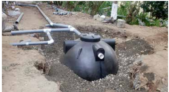
Above, left to right: In March 2016, MSD's David Glenn, Trish Capito and Steve Blanford traveled with WaterStep to install a septic tank in Orosi Valley, Costa Rica. Below, installation was underway.
