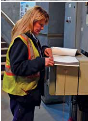
Floodwall Maintenance Electrician Patricia Capito keeps a watchful eye on operations at one of MSD's 16 flood pumping stations.
