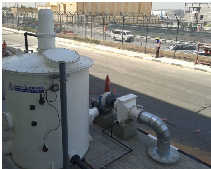
Figure 1 – Example Carbon Adsorption System
