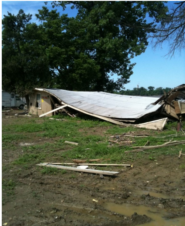
Home along Eifler Beach Road substantially damaged in 2011 Ohio River Flood
