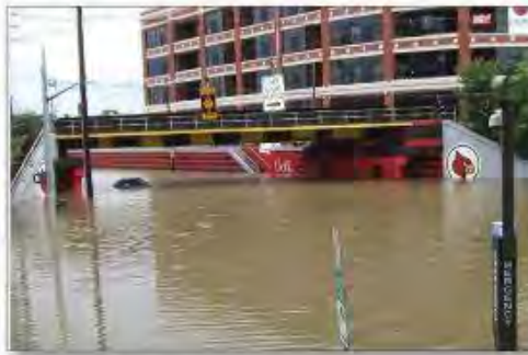
Viaduct at 3rd Street and Eastern Parkway after storm event
