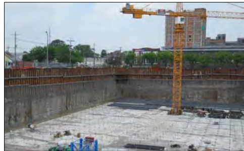
Logan St Basin Construction
