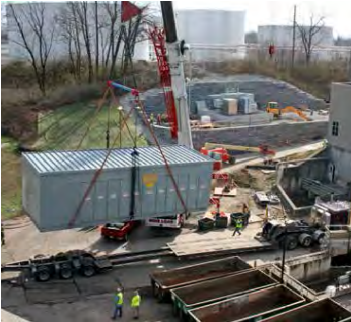
The new high-yard switch house is lifted from the transport truck bed.
