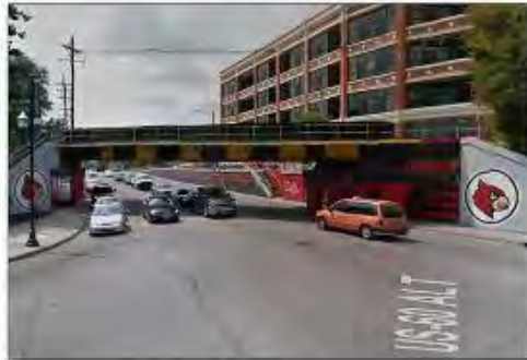
Viaduct at 3rd Street and Eastern Parkway before storm event
