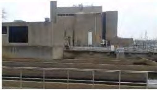
Morris Forman treatment plant prior to 2015 event
