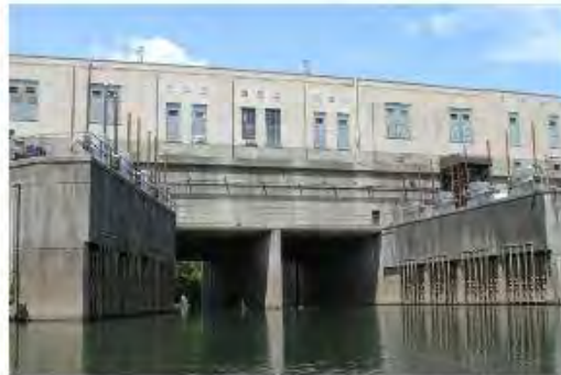
Beargrass Creek pump station
