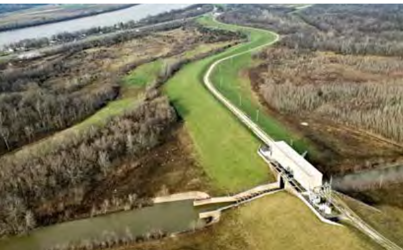
Pond Creek Flood Pump Station in southwestern Jefferson County
