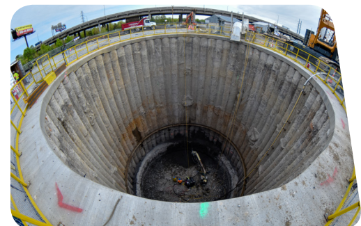
The tunnel-boring machine is expected to arrive in September 2018 and will be lowered into the tunnel in pieces and reassembled for operation. It will dig a tunnel 20-feet in diameter and approximately 200 feet below the surface, which is more than 18 stories below ground.
